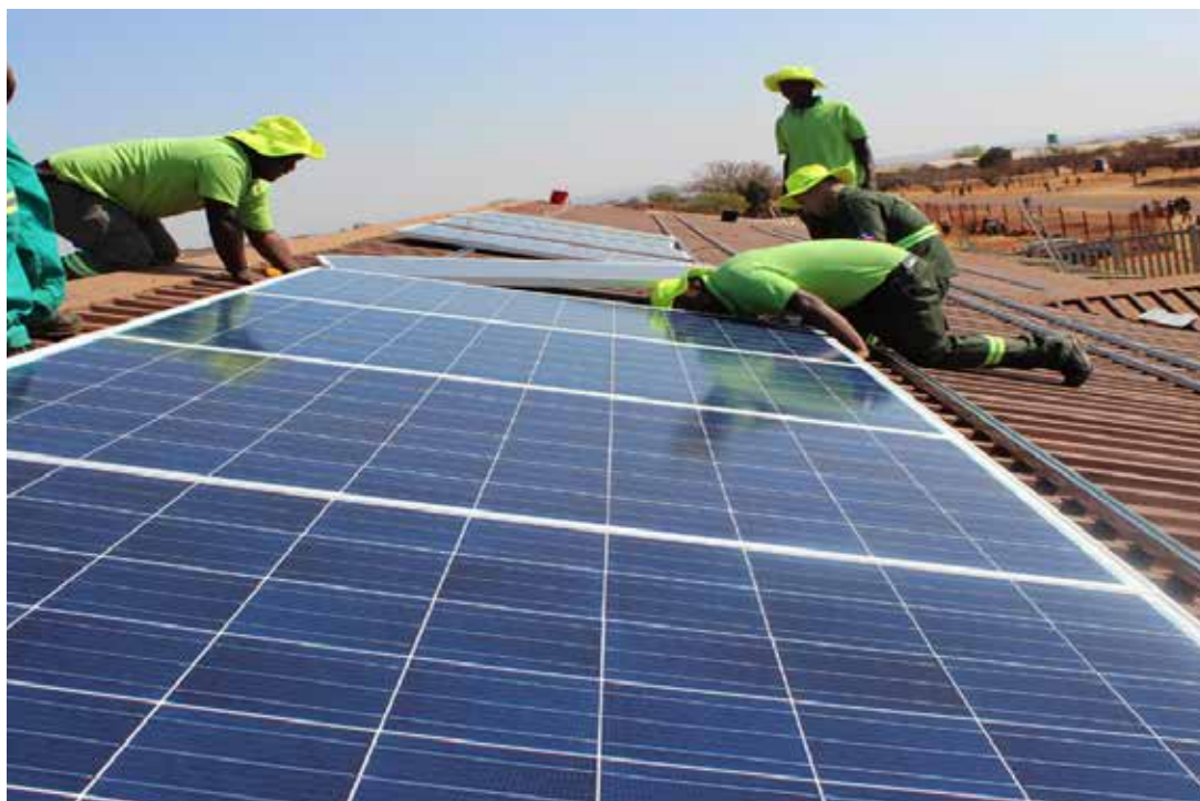
Installation of solar panels in South Africa
